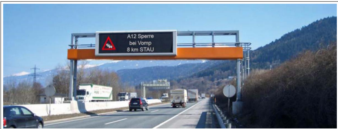
Figure 16: Dynamic message sign as part of the traffic management system at the A12 freeway in Tyrol
