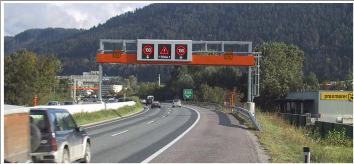
Figure 15: Variable speed limitation as part of the CCS at the A12 freeway in Tyrol
