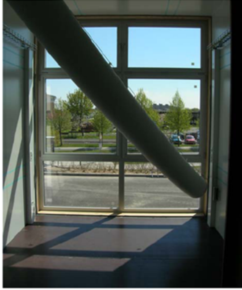
Figure 3.6: Air distribution hose [3]
