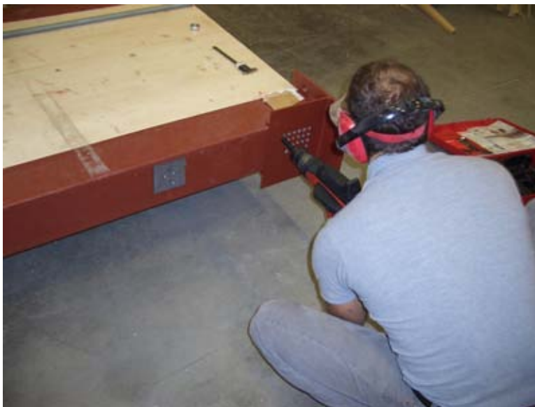
figure 6.10: Connection for high tensile force anchorage made by Hilti-nails
