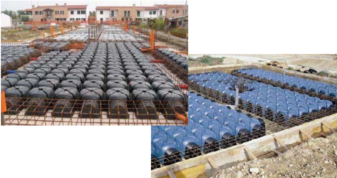
Standard Italians Polypropylene elements for crawl space – Pontarolo engineering Pordenone (Italy)
