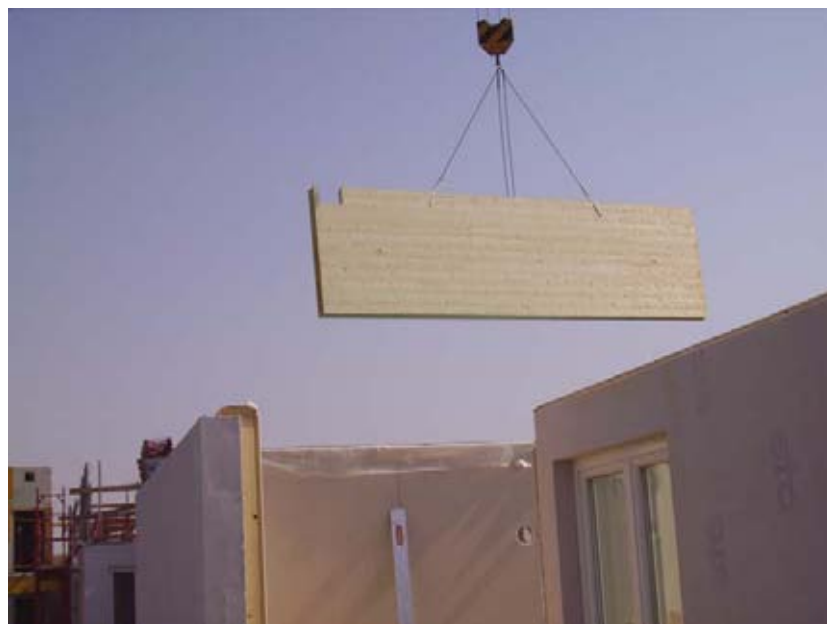
Wooden panel structure of a multi storey passive house – Vienna 19 th July 2007 - 36,7°C
