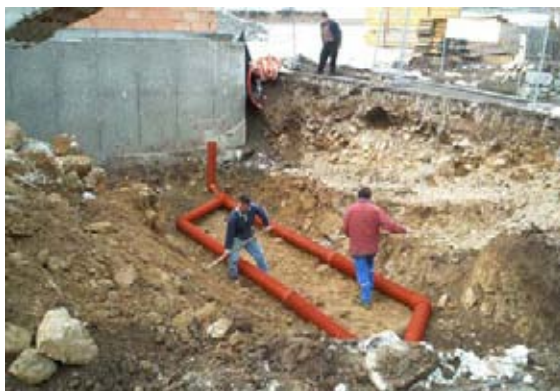
Subsoil heat exchanger system during summer time
