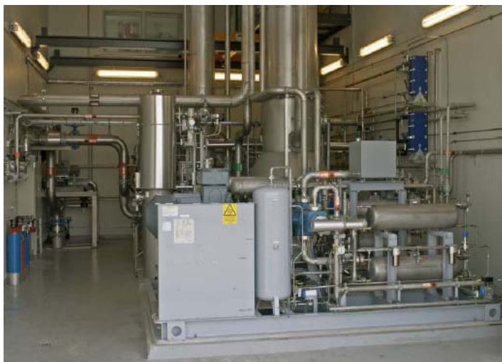
Picture 3: 600 m 3 /h upgrading plant with water scrubbing technology – Henriksdal sewage plant, Stockholm (Jönsson)
