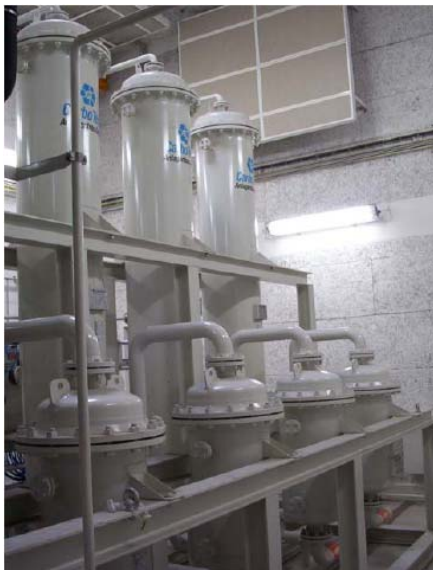
Picture 2: 350 m 3 upgrading plant with PSA technology - Helsingborg, Sweden (Jönsson)
