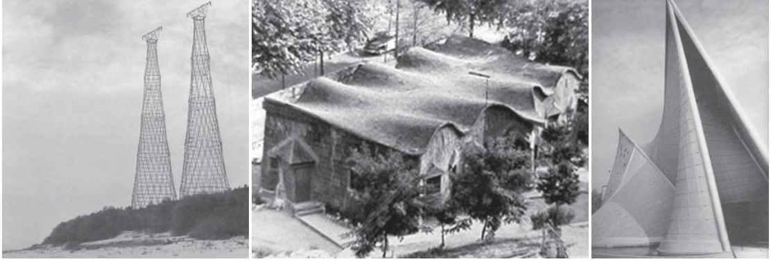
Figure 6.7: Ruled surfaces in architecture: An electricity pylon by Vladimir Shukhov, the roof of the Escoles Sagrada Família by Antoni Gaudí and the Philips Pavilion by Le Corbusier and Iannis Xenakis (from left to right, photo credits: Igor Kazus, Carlos Martínez, (Jencks, 2000)).
