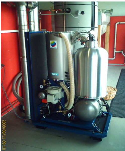
Picture 8 43 : Sunmachine Pellet with puffer tank
