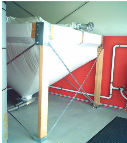
Picture 9 44 : Textile silo for Sunmachine Pellet
