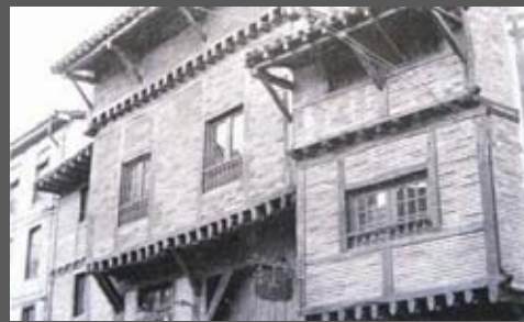
Figure 4.2(d) Use of timber framing in urban areas
