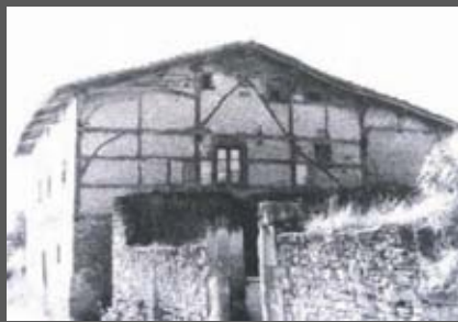
Figure 4.2(c) Timber frame on the upper floor
