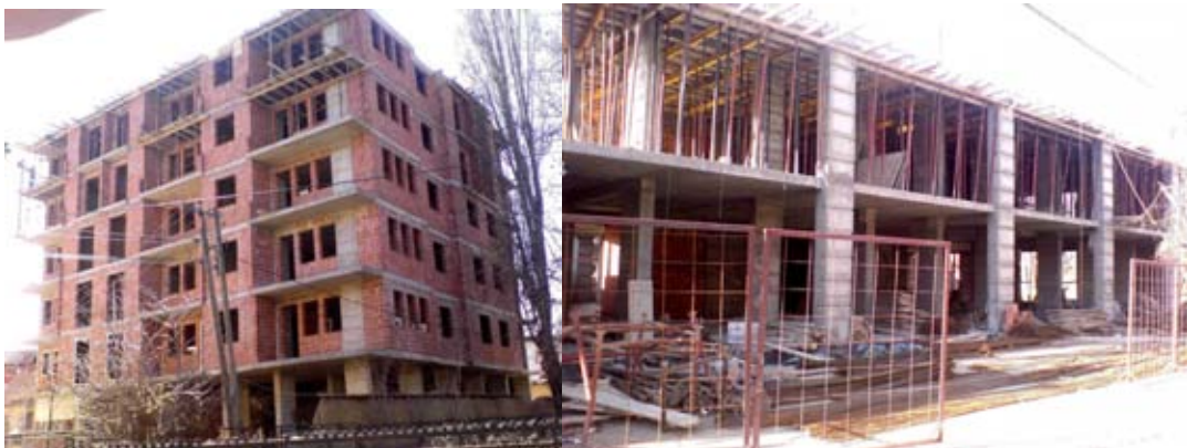
Figure 4-1: Reinforced concrete structure of residential buildings
