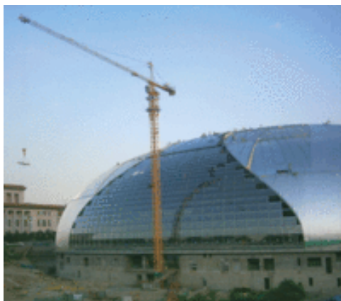
Fig.6.8: in Beijing, China's National Opera Hall features self-cleaning glass coated with a film of photocatalytic nanoparticles that can break down dirt.
