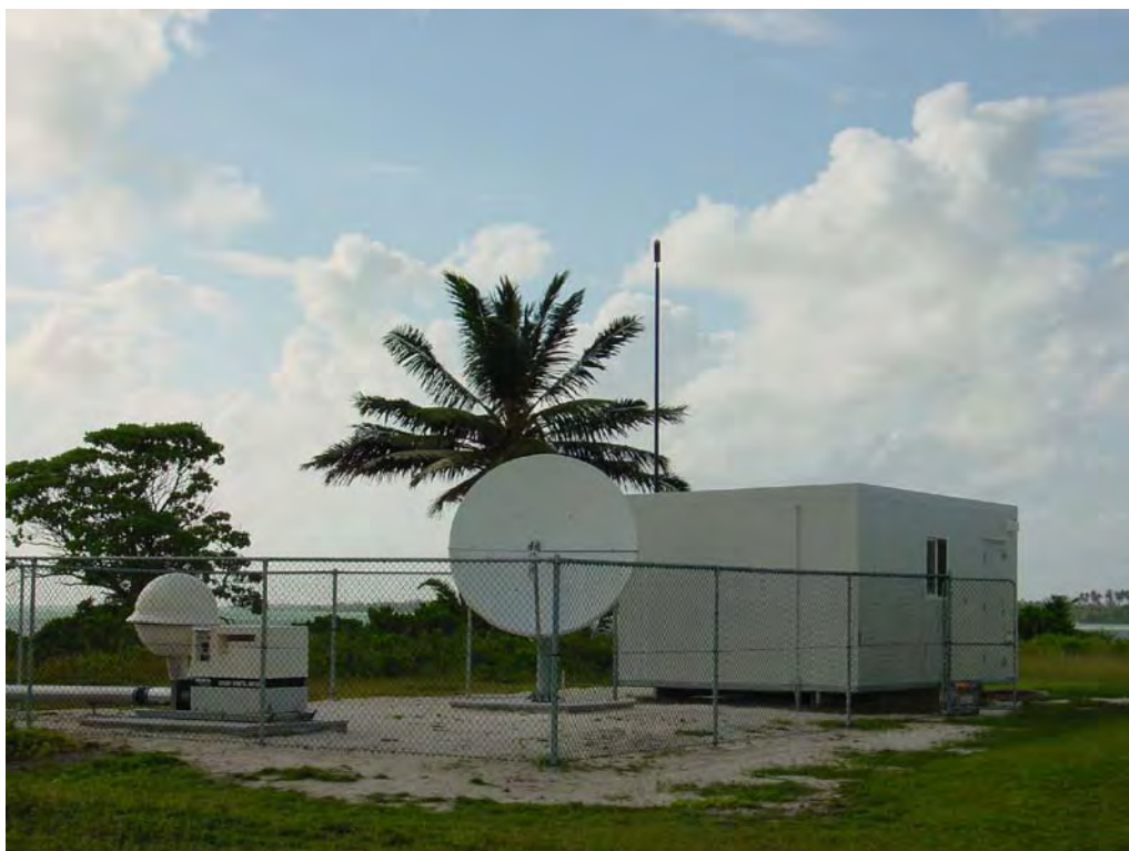
Figure 11 Typical Radionuclide Station Layout. Sampling system on the left, satellite communication system in the center and detector room on the right
