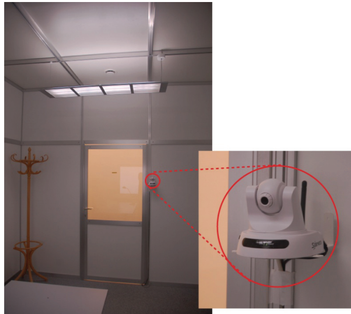
Figure 4-6 The installation of IP Camera
