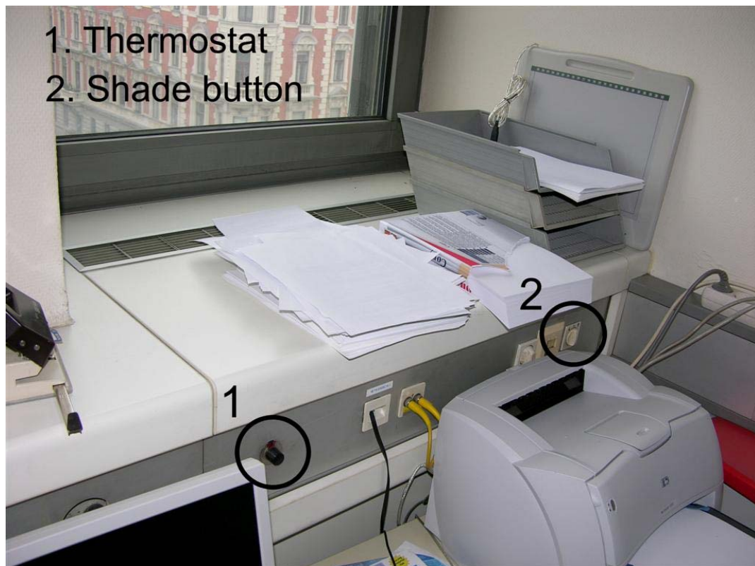
Figure 109 View of the buttons for manual control of shading and fan coils in the FH office
