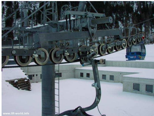
(c) A holding-down sheave assembly.
