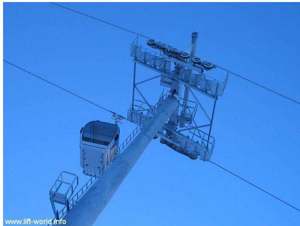
(a) A tower with a carrying sheave assembly.
