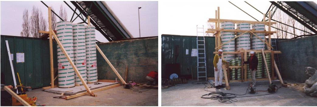
Figure 8.4: Construction of the formwork.
