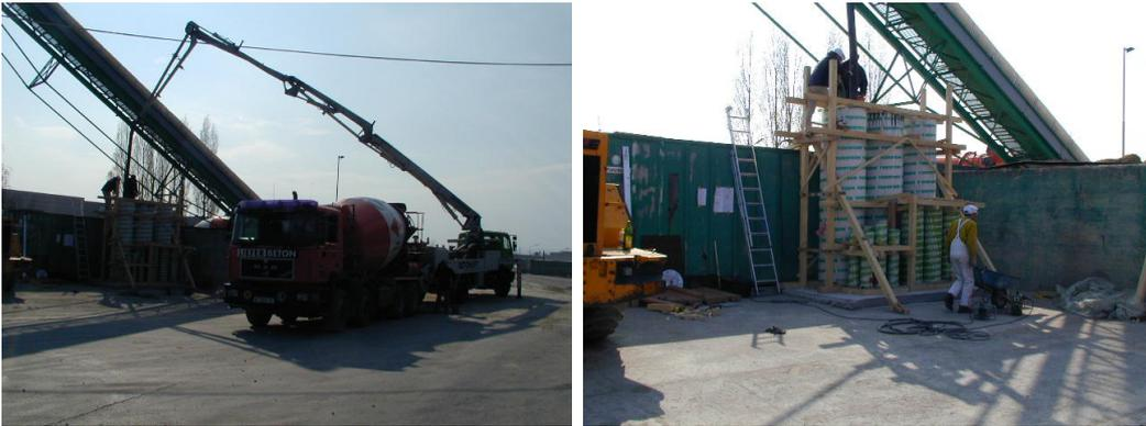
Figure 8.6: Producing the specimen with the concrete pump
