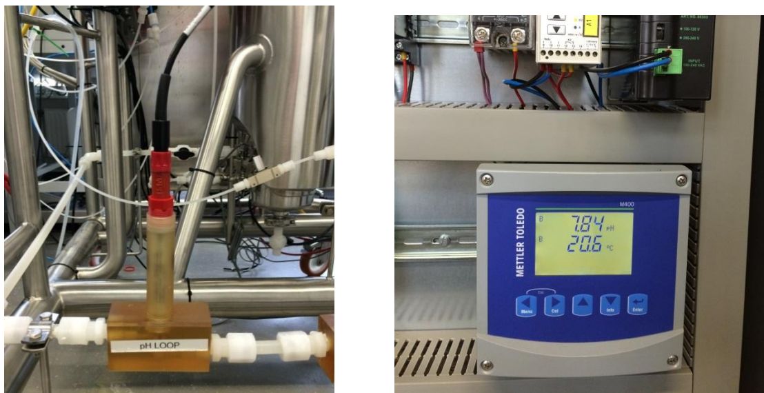
Figure 49: pH-Probe in Loop and pH-Transmitter in Switchboard
