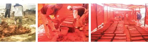
The wall: As the walls are only self-load bearing a single bond of one row of headers and one row of stretchers was used (see fig. 200). For the arches and the vault a brick size of 25 x 25 x 25cm was used.
