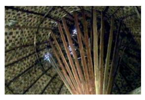
fig. 204: Holes in the bamboo roof of Adena SRDU
