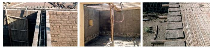
fig. 95: Ring beam with reinforcement before filled up with concrete
