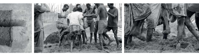
wall, the more difficult it is to execute with adobe bricks. If the wall is e.g. thicker than 60cm, a lot of material will be needed and it would take a long time to lay all the bricks, so it becomes less economical. In this case, a different construction like a cob wall or a rammed earth wall may be better. (Houben/ Guillard 1989)
