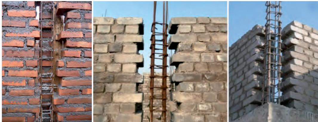
18 - „Tothing applications: a) recommended construction practice (S. Brzev) with horizontal reinforcement“ (GSDMA 2013)
