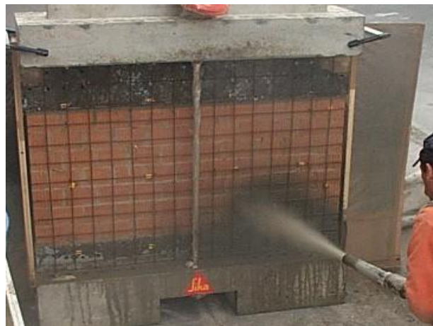
Figure 6-2 Applying Shotcrete
