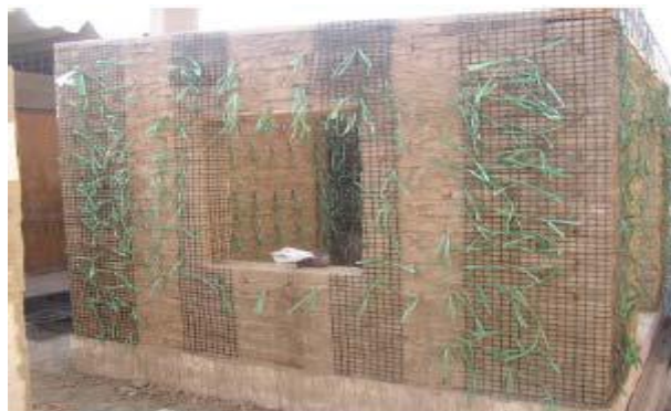
Figure 2-14 External geogrid mesh reinforcement
