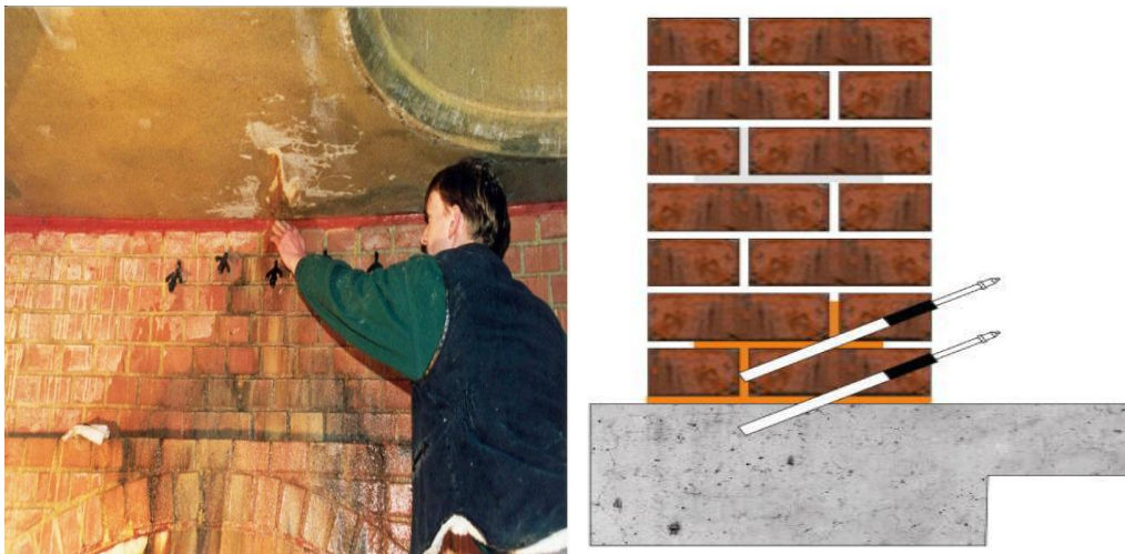
Figure 6-5 Applying the injection method to an existing masonry brick wall
