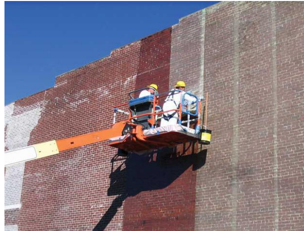
Figure 6-3 FRP retrofitting method
