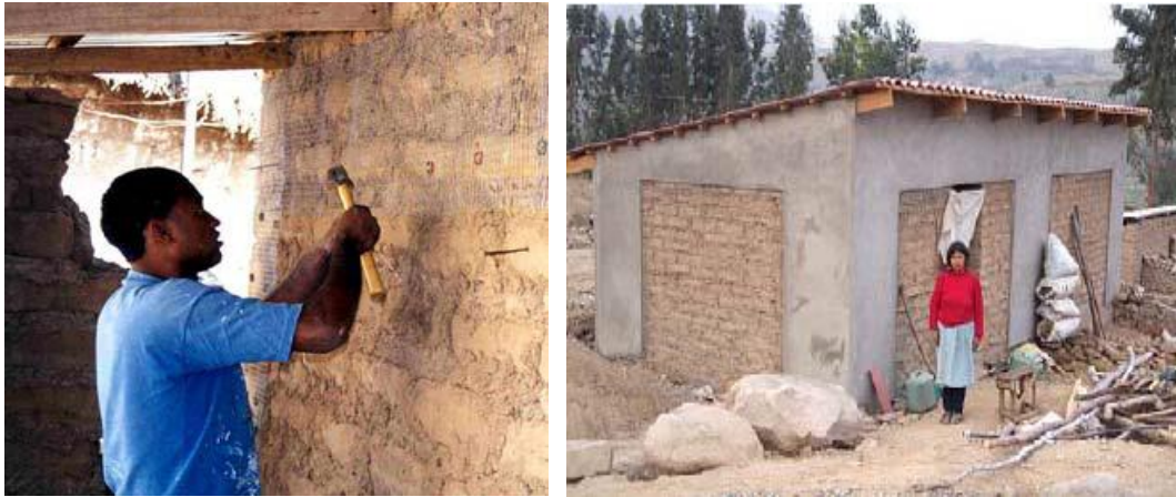
Figure 2-13 External wire mesh reinforcement introduced by Marcial and Rafael
