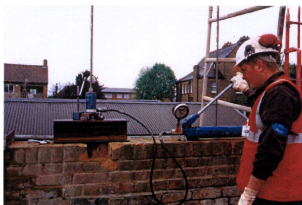
Figure 6-4 Applying post-tensioning method
