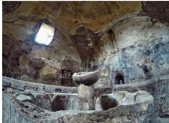
Fig. 46 (middle-left) Gazi Ali Bey Hamam, public bath built in the late 14th century, Vushtrri
