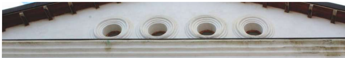
Fig. 169 Close-up image of facade details of Haxhi Zeka Mill, Peja, Peja
