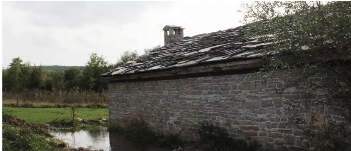
Fig. 161 Rear view of the Old Mill of Banja, Banja, Malisheva
