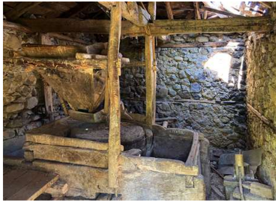
Fig. 108 Grinding mechanism at the Mill of Biçec Village, Biçec, Kaçanik
