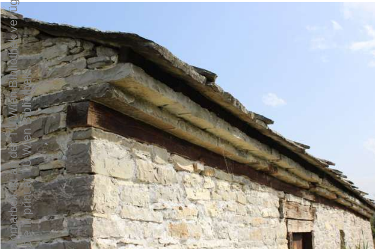
Fig. 90 (left) Close-up image of the stone slab eave at the Old Mill in Banjë, Malisheva
