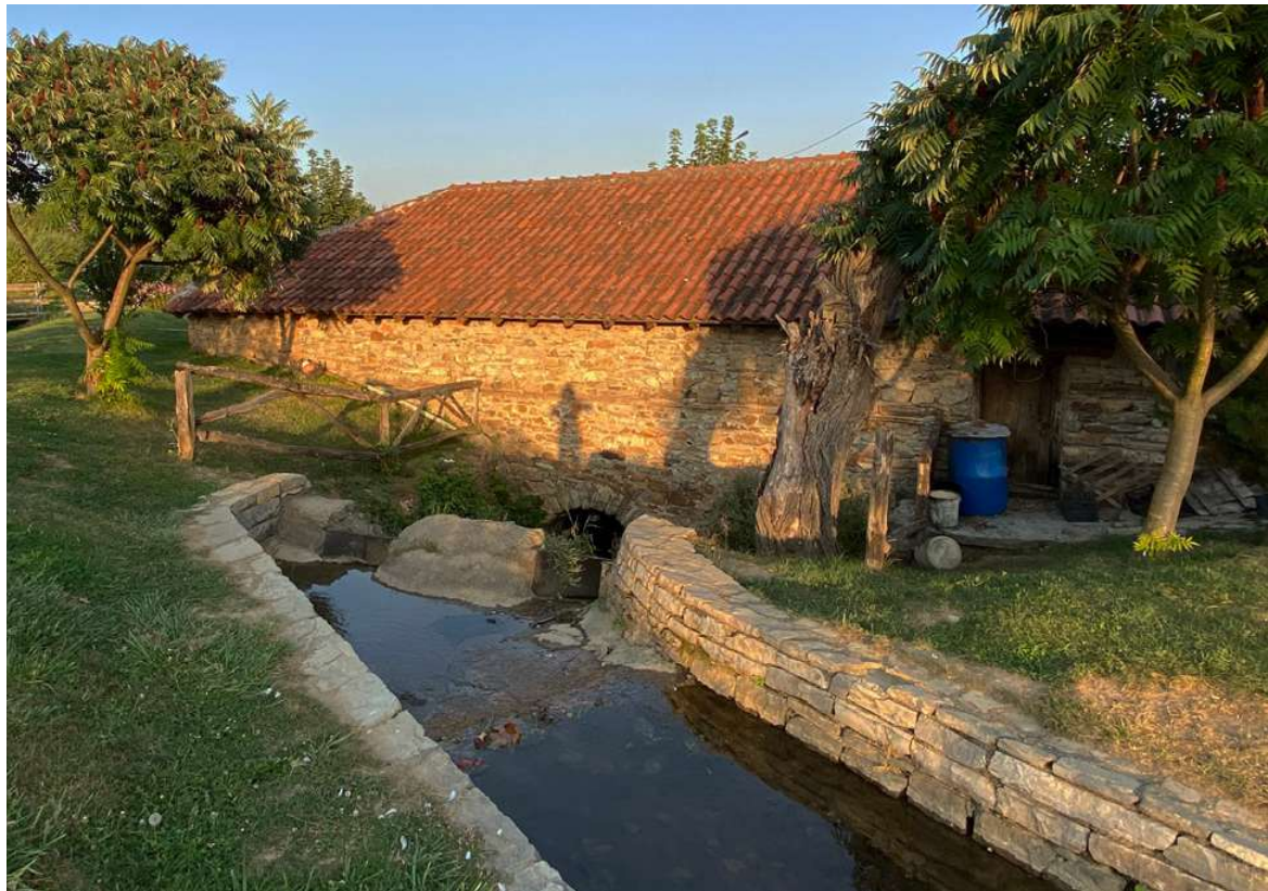
Fig. 179 Back view of the mill - water dam, chutes and the mill arch, Mill of Nika, Ferizaj
