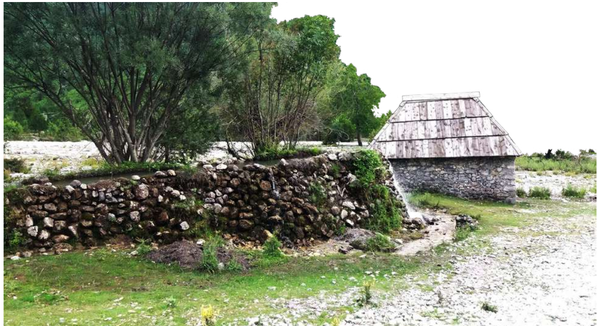
Fig. 28 The dam built by stones and the mill building, Watermill of Ndërlyhaj, Theth, Albania
