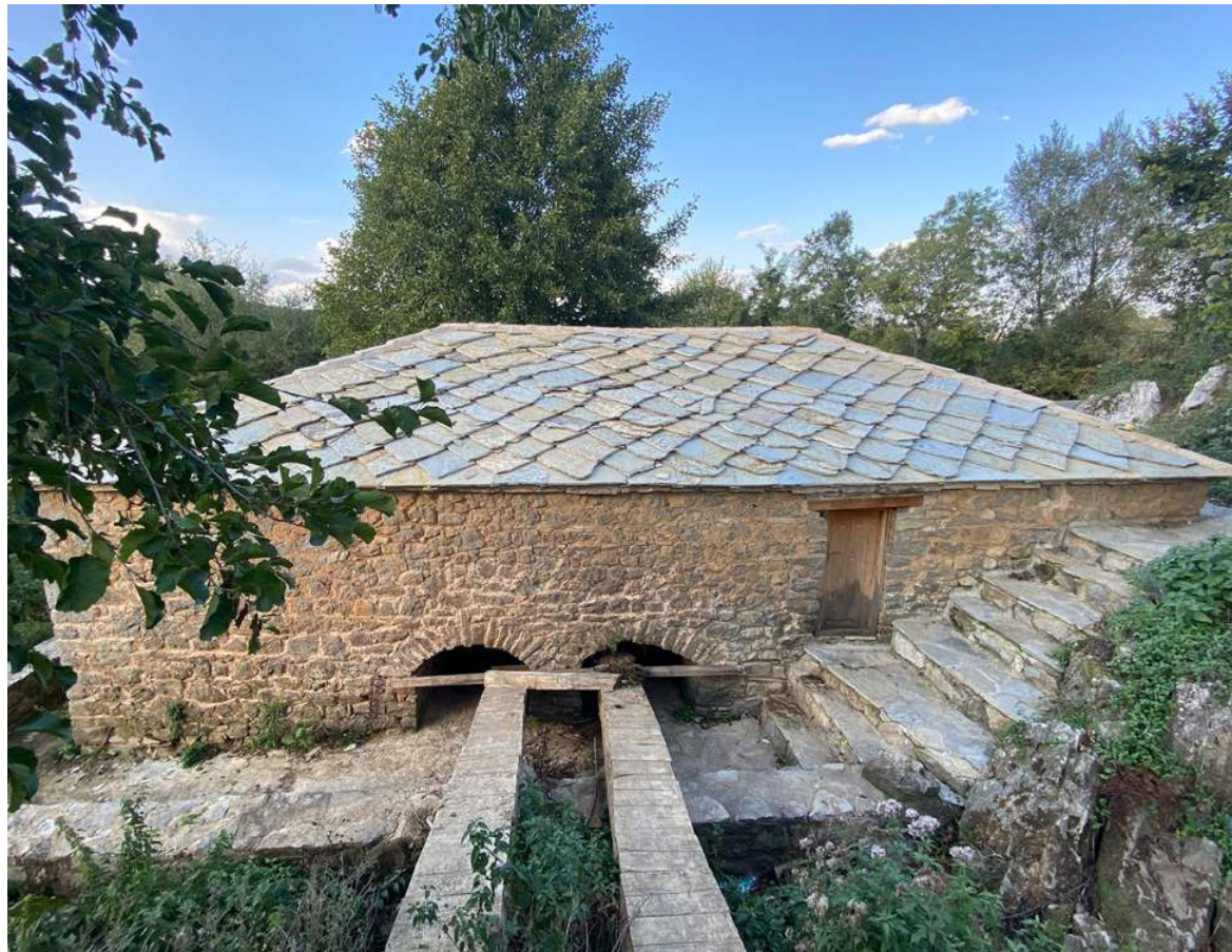
Fig. 145 Mill of Rexhep Shatri The rear side of the building, mill arches and chutes
