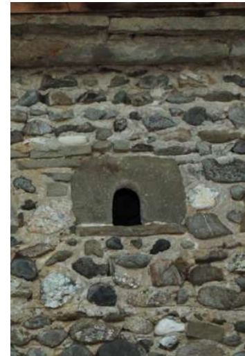
Fig. 100 Rectangular window with monolithic stone frame at the Mill of Tahirsadriaj family, isnqi, Deçan
