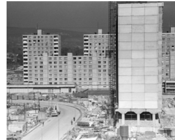
Fig.15 Construction site Fedinova street
