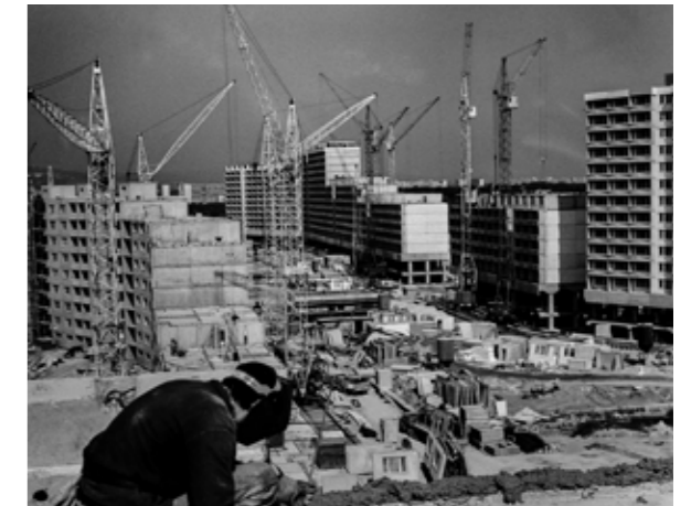
Fig.16 Construction site Petržalka
