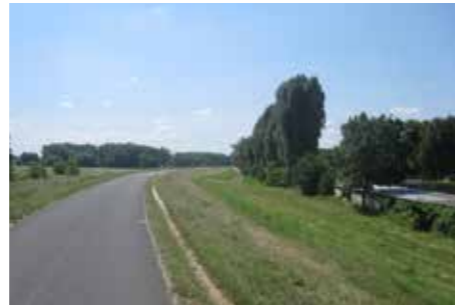
Fig.81 Flood protection dam
