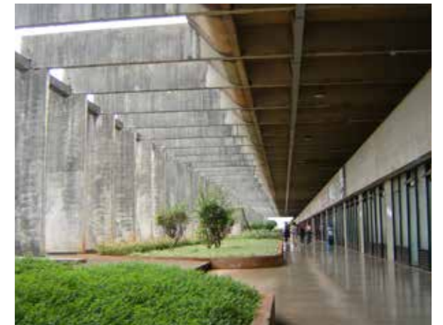
Fig.88 Perfect harmony of green and concrete
