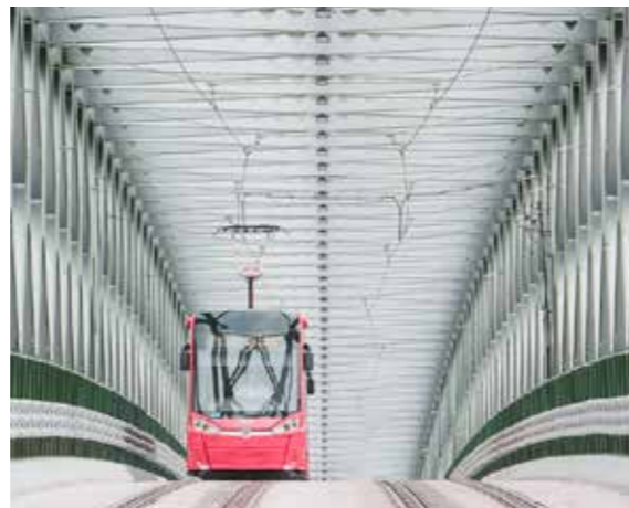
Fig.50 Old Bridge newly reconstructed - specifically for trams
