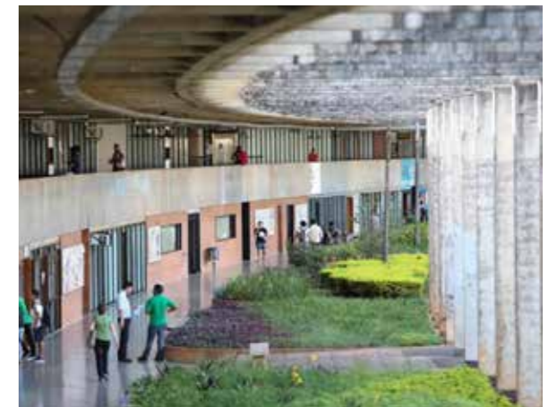
Fig.87 View from second floor
