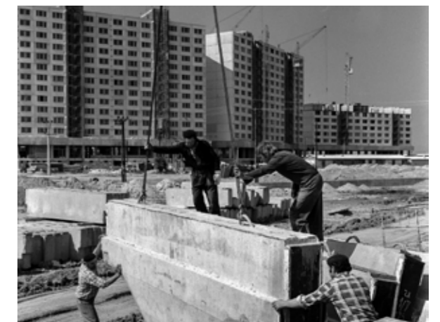
Fig.18 Construction workers lifting a concrete panel
