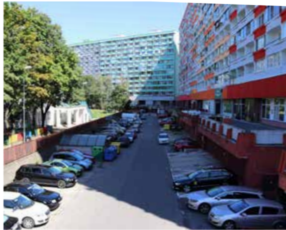
4. Different height between the flats ground floor make a complicated connection between residents and amenities
