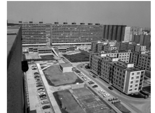
Fig.22 View from a roof
