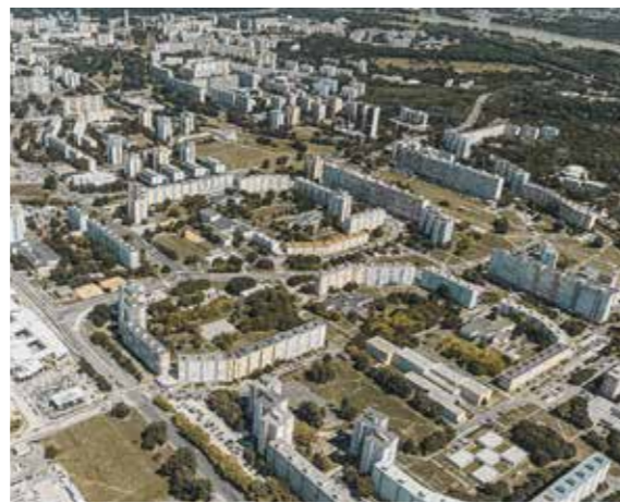
Fig.55 Aerial view prefab buildings
