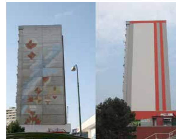
Fig.98 Old vs New facade
