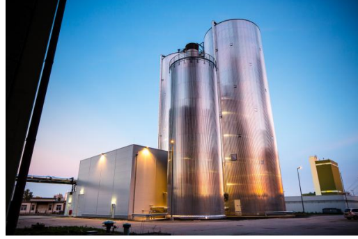
Figure 1.4.: Picture of the of the storage tanks ©Wien Energie/EHM
