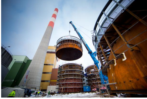
Figure 1.3.: Construction of the storage tanks ©Wien Energie/EHM
