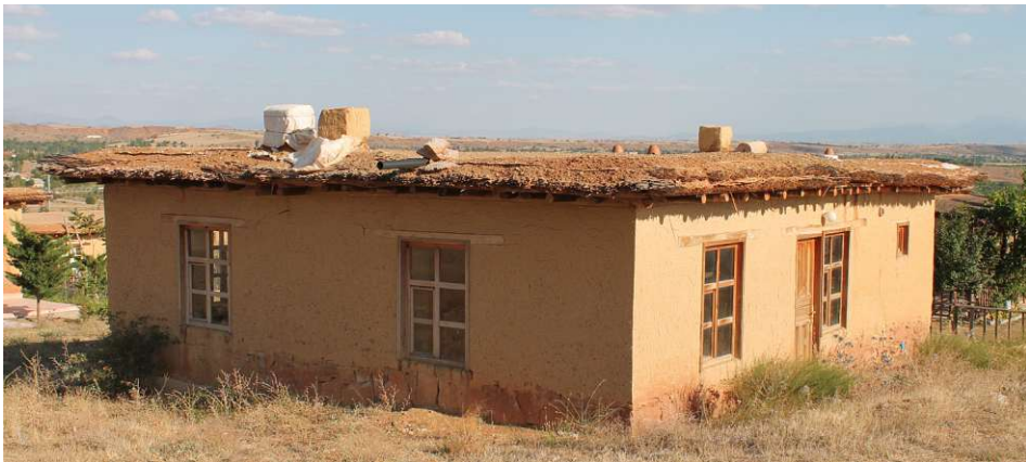
Abb. 82: Lehmhaus in Sonsuz Şükran
